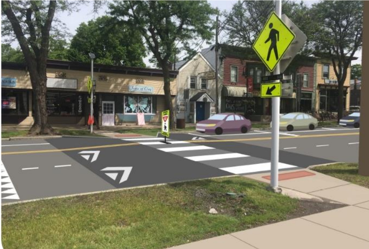
Image 1 – Example of a Raised Crosswalk (and RRFBs) with Pavement Markings
